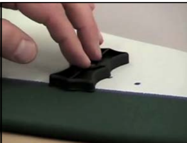
Set liner attachment in marked location.
